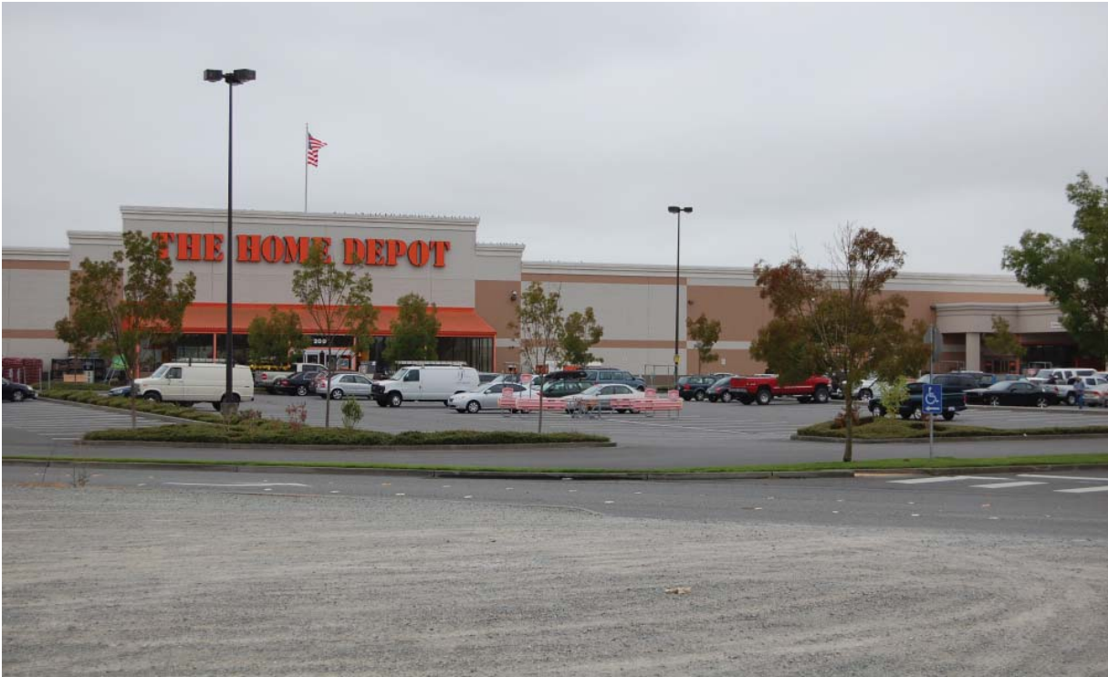
Existing conditions of Home Depot in Burlington, WA.
