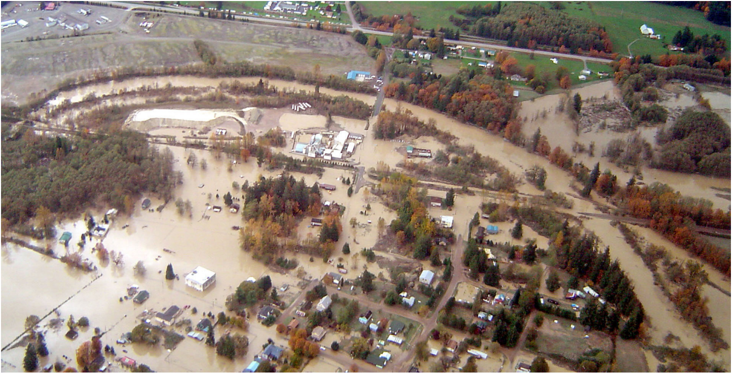
Town of Hamilton Flood, 2003
